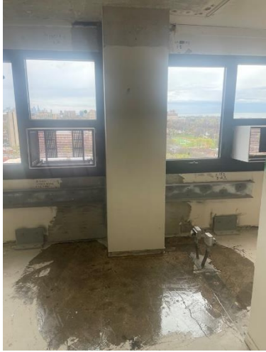
Epoxy coating of cracks
